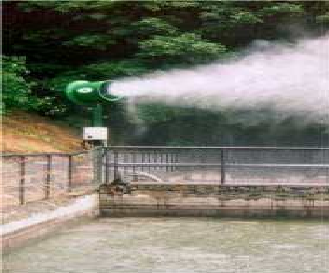
Figure 3. A typical atomizer installation for odour control
